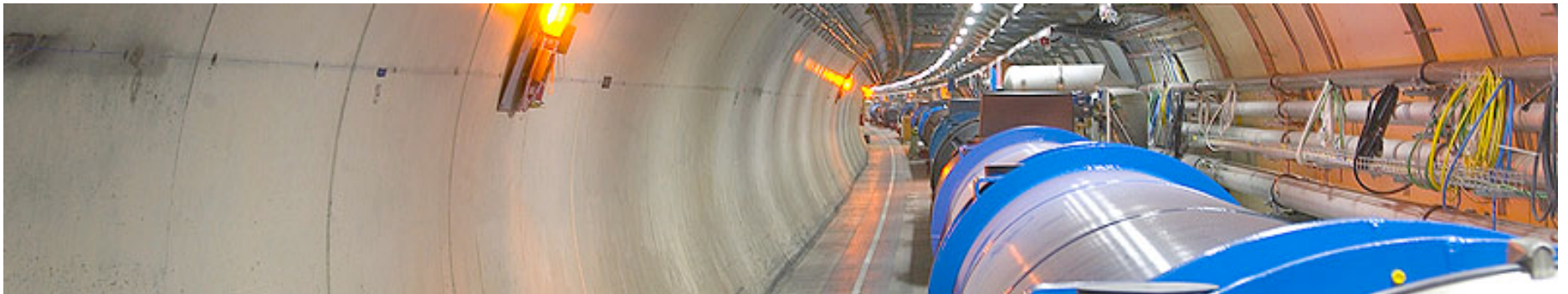
2008 – all ready for beam
