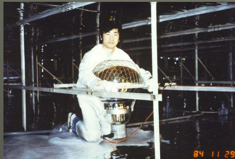
Installation of bottom anti-counters.
