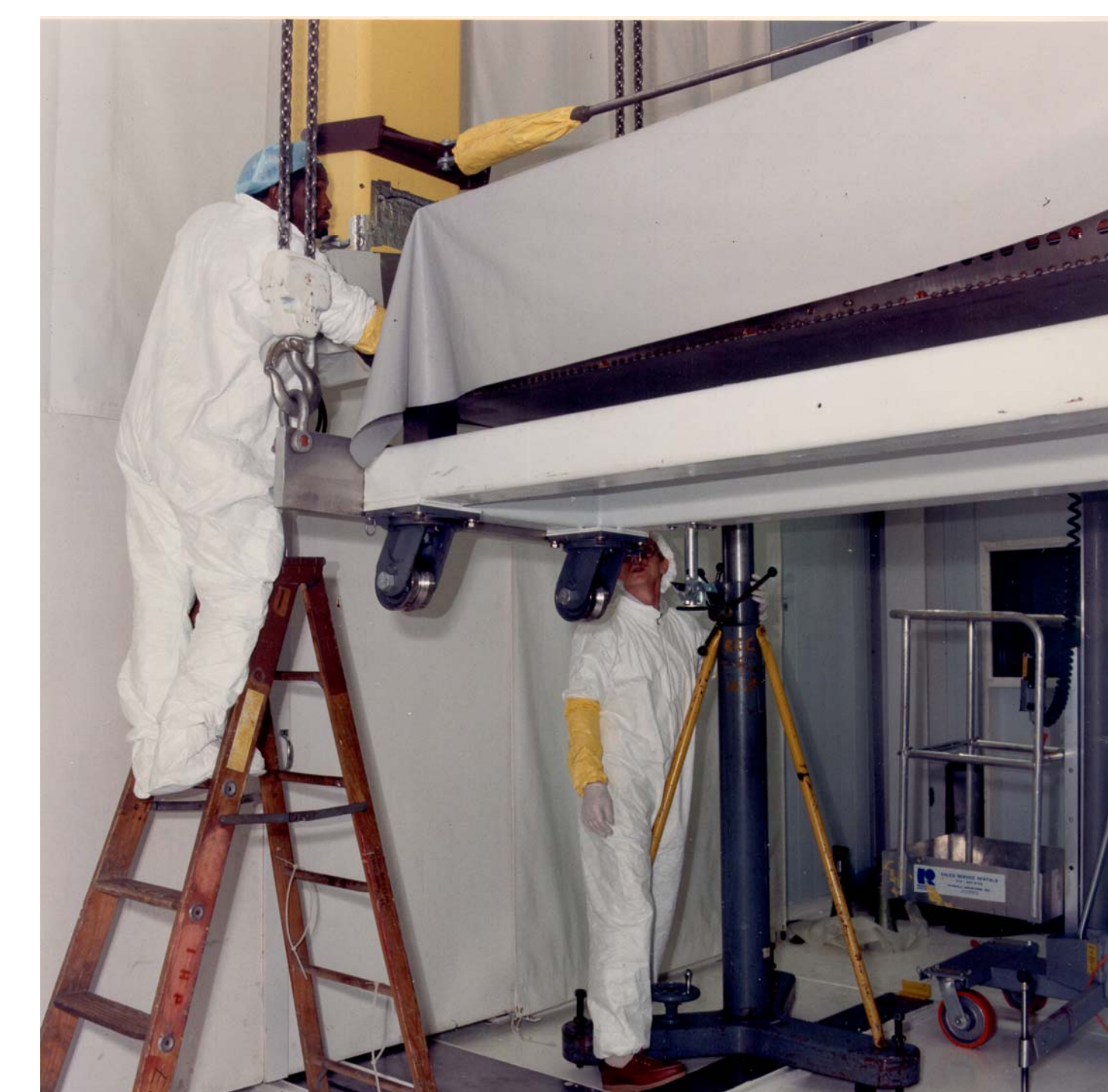
Putting a module on the C-frame for installation
