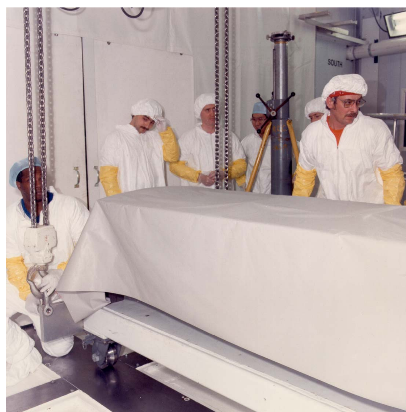
Preparing to lift a module onto the installation C-frame
