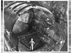
Water tank used for shielding around neutrino experiment in Homestake mine (4850ft) by Ray Davis (in photo)
